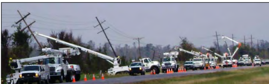
Hurricane Gustav Storm Work
