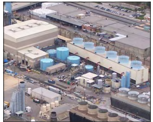
Magnolia Power Plant
